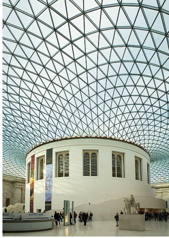
FIGURE 2.1. Lattices spanning the roof of the Great Court of the British Museum, London.
